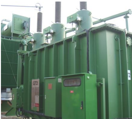
132 kV Natural Ester Filled Transformer, UKPN
